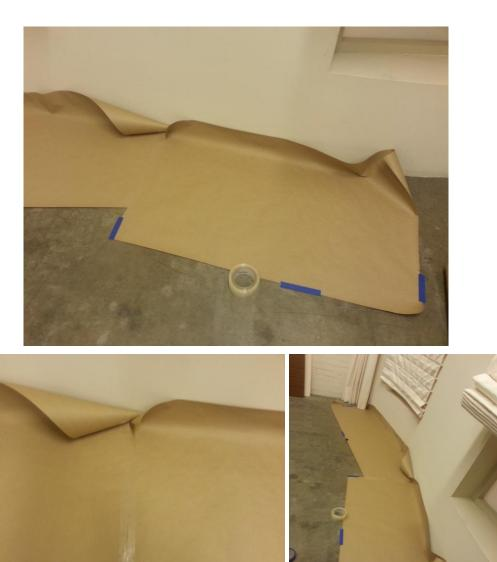
**Note**: Often the shape of the area to be templated exceeds the depth and length of the paper. If so, splice on a piece of kraft paper. Be sure to tape the splice on both sides of the paper so it doesn't pull apart.
